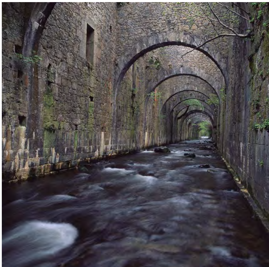
Figure 14.3: The arms factory in Orbaizeta (Navarre, Spain) is one of the many places where rivers were harnessed to use hydraulic energy. Most streams and rivers were thus dammed and channelized
