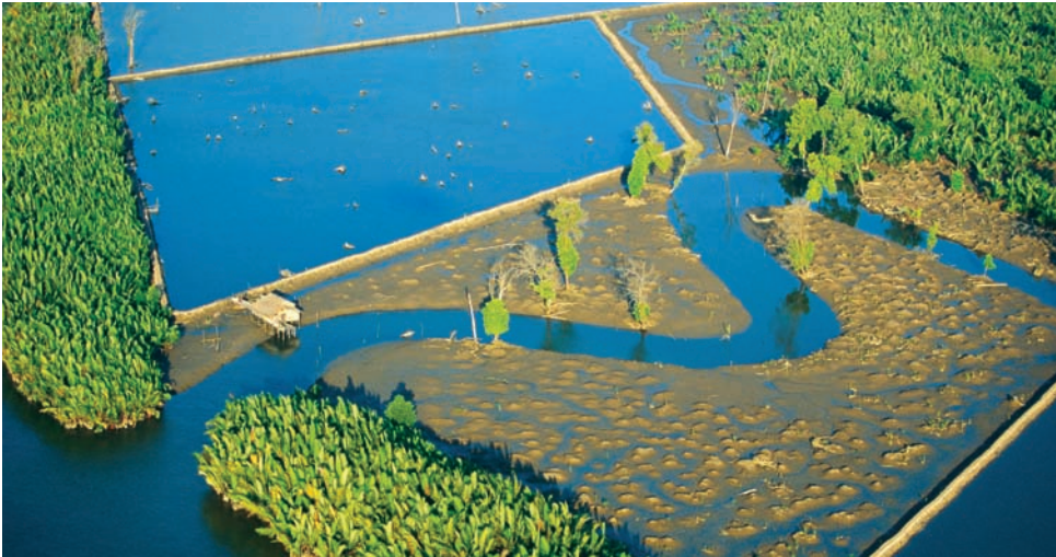
Photo 4.6: Bornean mangrove forest. This aerial view shows dykes and enclosed shrimp ponds carved out of the mangrove habitat.
